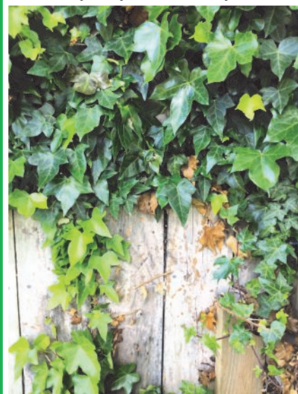
Ivy penetrating a garden fence.
